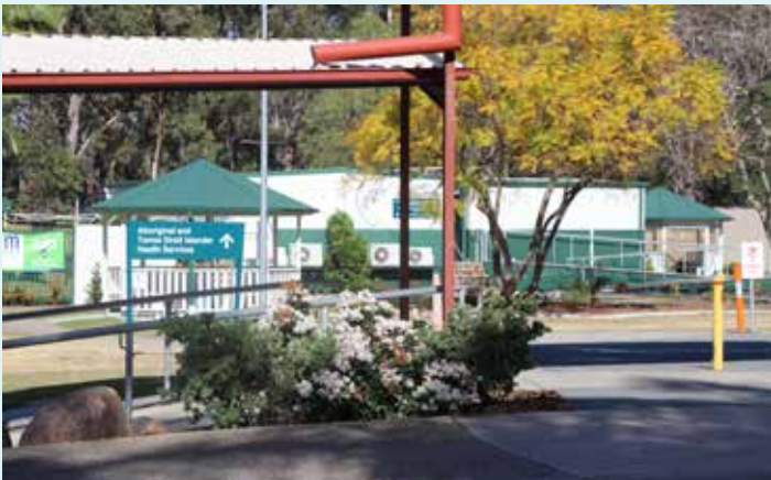
The demountable is located at Building 23 on the hospital campus (next to the TPCH pool).
