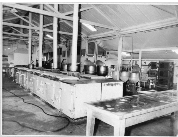
MAIN KITCHEN IN EARLY DAYS WITH COMBUSTION TYPE STOVES
