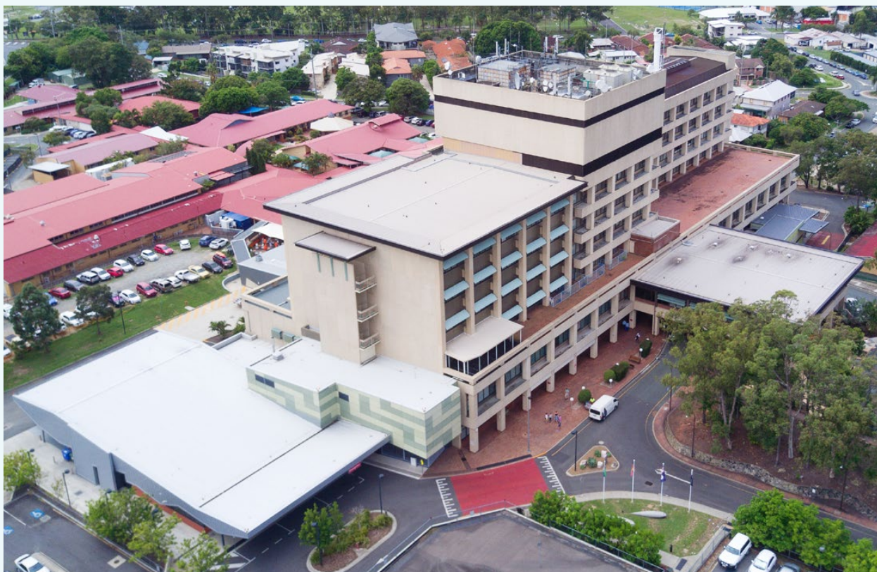
A renewed and refurbished Redcliffe Hospital will continue to serve the Peninsula for decades to come.
