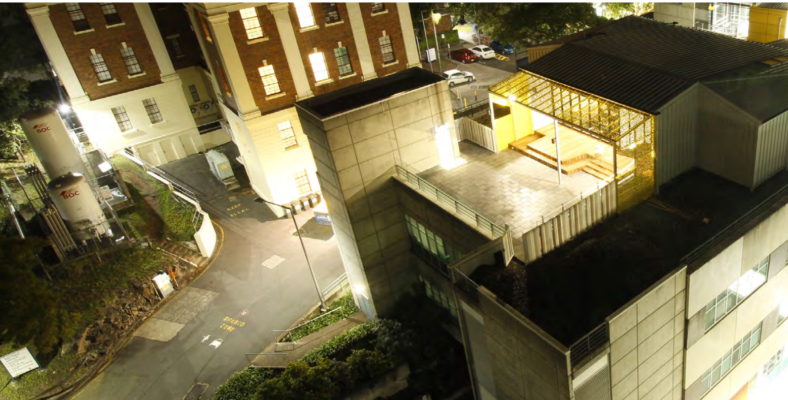
Sony Foundation's rooftop You Can Centre at Royal Brisbane and Women's Hospital.
